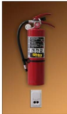
One of the most important things about a fire extinguisher is to make sure there is enough pressure in it to operate. This is often indicated by a small gauge near the handle. Usually, an arrow will either point to a green area (enough pressure) or a red area (not enough pressure in the extinguisher).
